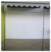
9. Position the footplates and lower down the telescopic supports onto them.
