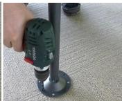
11. Mark the location of the footplate's mounting holes and then drill holes for pins or anchors fixing the support.
