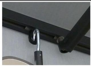
3. Insert the support's hook into the eyelet bracket mounted to the awning's front bar. Repeat this step for the second support.
